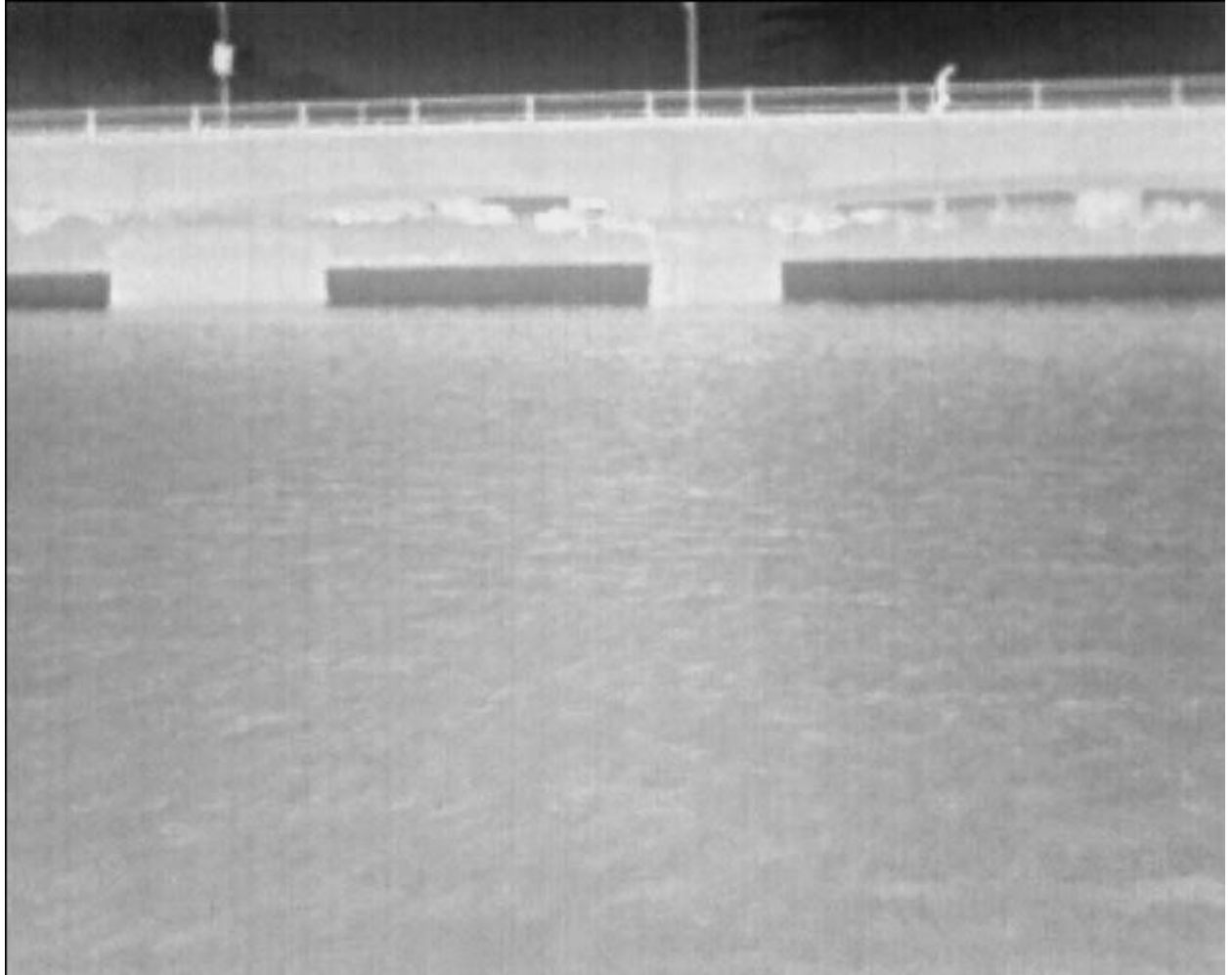
Image from REx - (IR) Harvard Bridge, abutments, pedestrian
