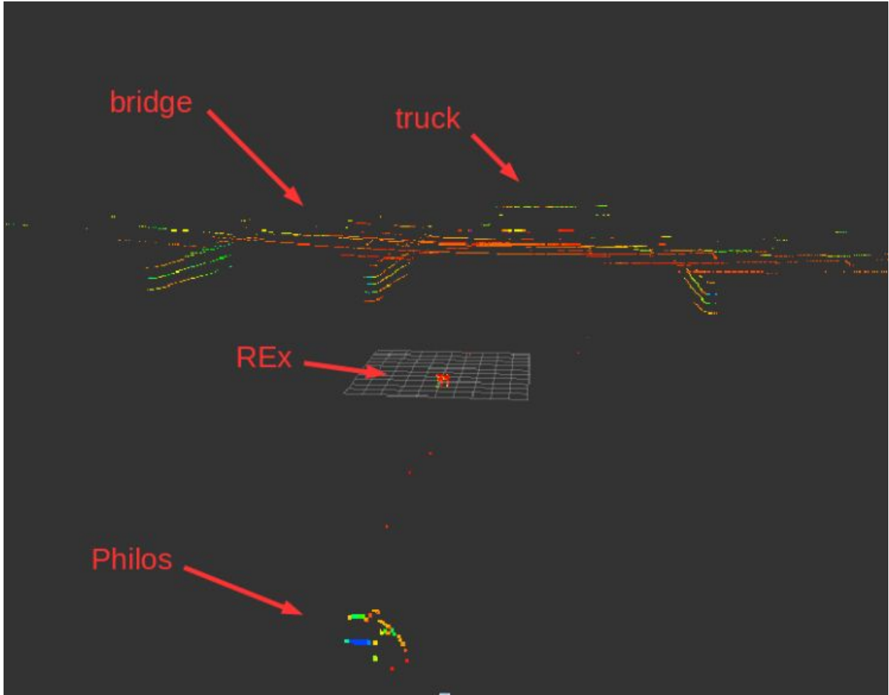
Images from REx (cloudy): (LIDAR) Harvard Bridge, annotated
