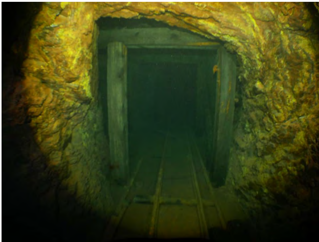
Figure 84. Image of the mine's drift supported by beams. The small gauge rail can be seen running along the floor and a candle holder is still attached to the right wooden beam. (Leah Potts)
