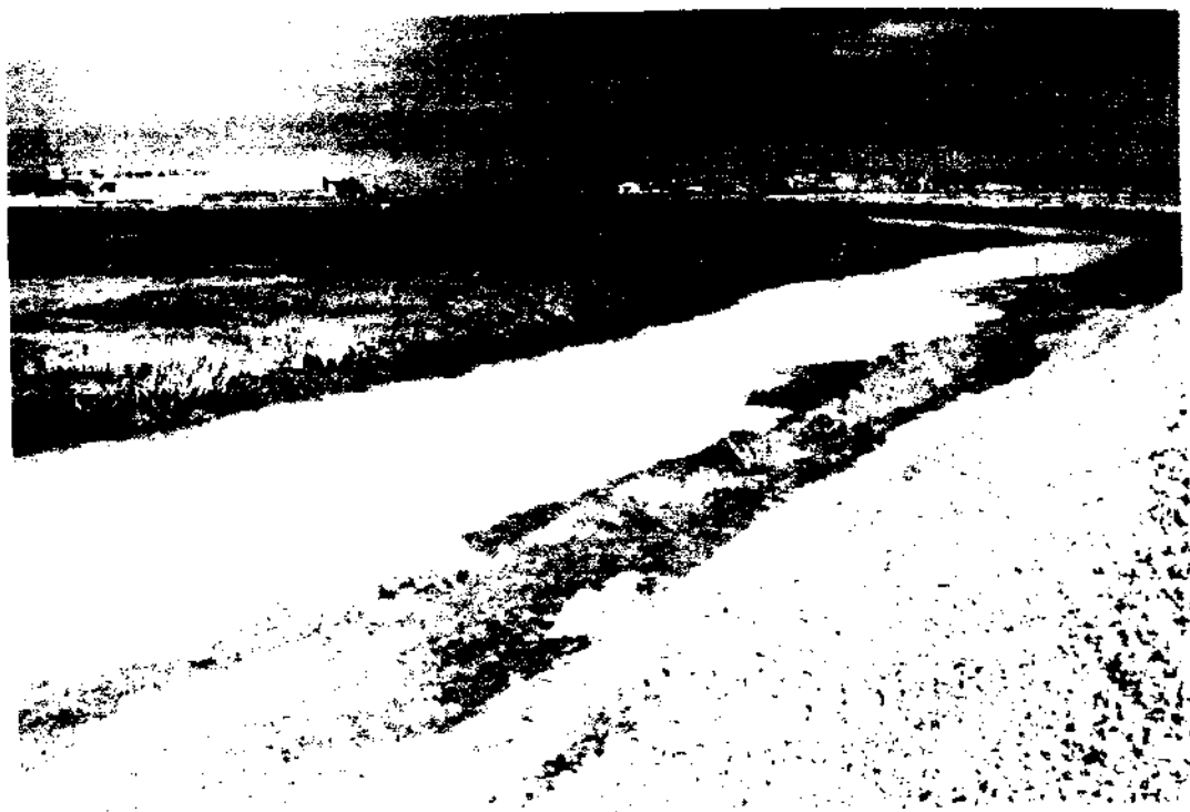
Figure 3: Channel excavated by dragline from a dike at Muzzi marsh, Corte Madera, CA
