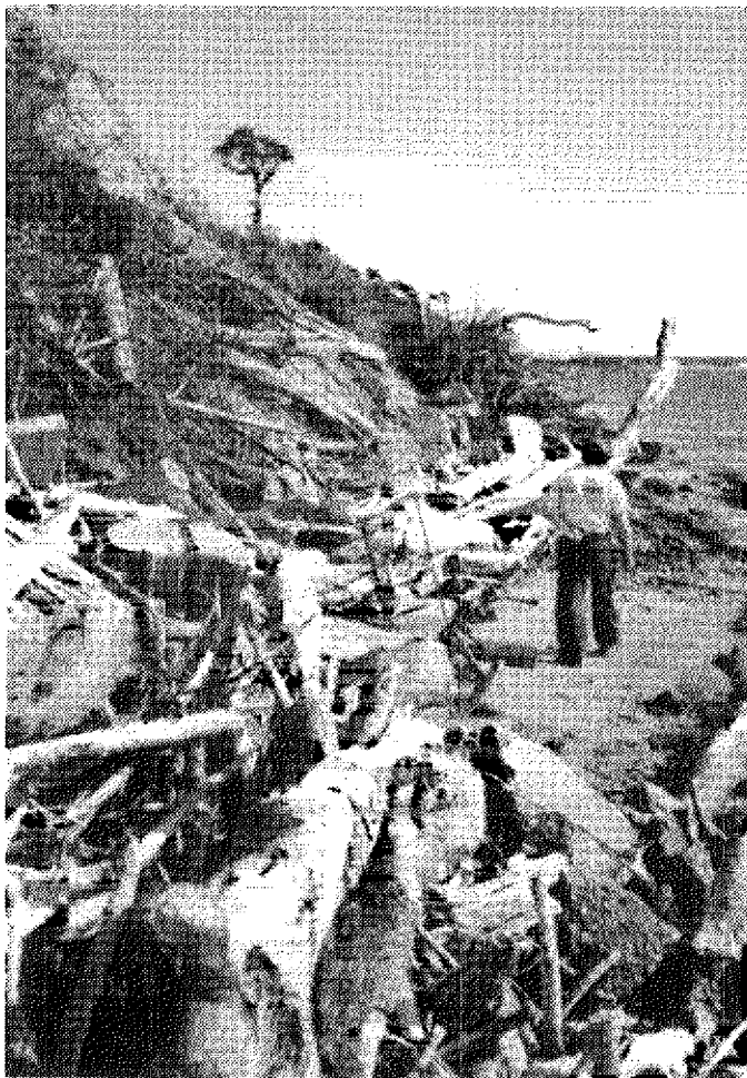
Fig 39. Dead wood dumped at bank toe to dampen wave energy
