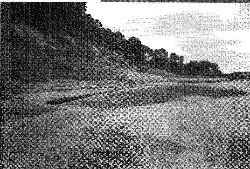
Fig 5. Bio-engineering (bio-logs and vegetation) in a low-wave energy environment
