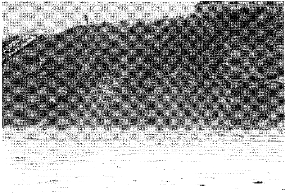
Fig 28. Coastal bank with fill and jute netting being planted
