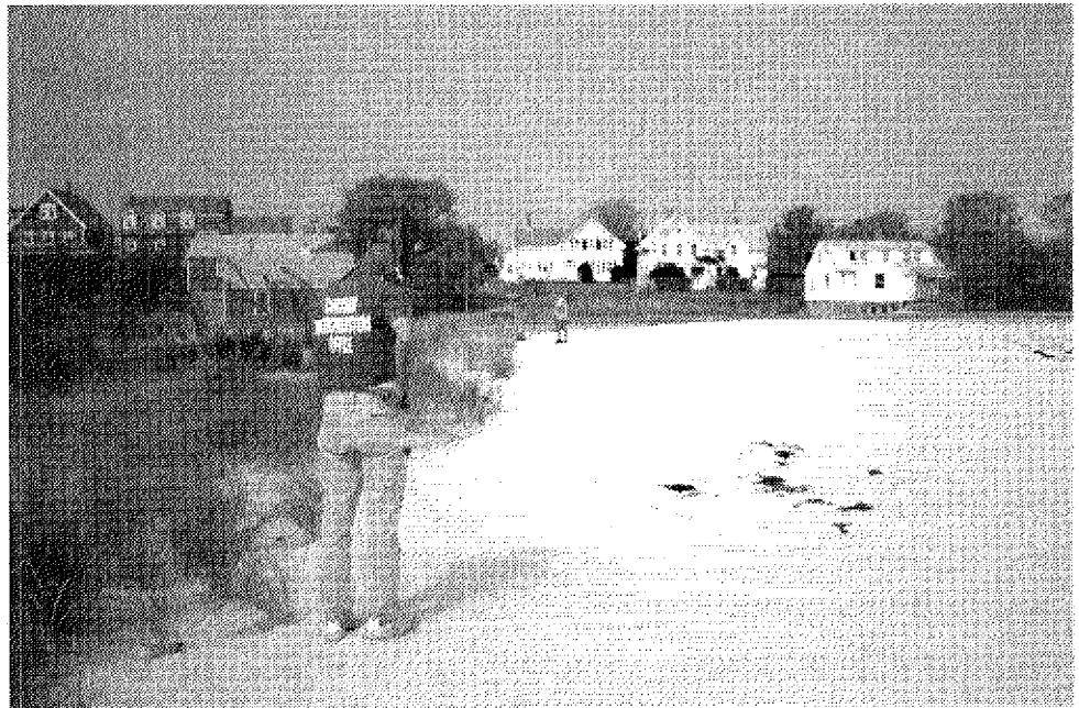
Fig 21. Preparing the dune restoration site in Chatham
