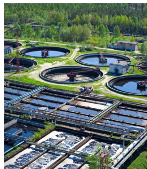
Photo: Water Treatment Plant, Antiksu
