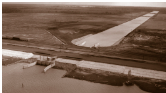
Davis Pond freshwater diversion structure. Photo courtesy of U.S. Army Corps of Engineers.
