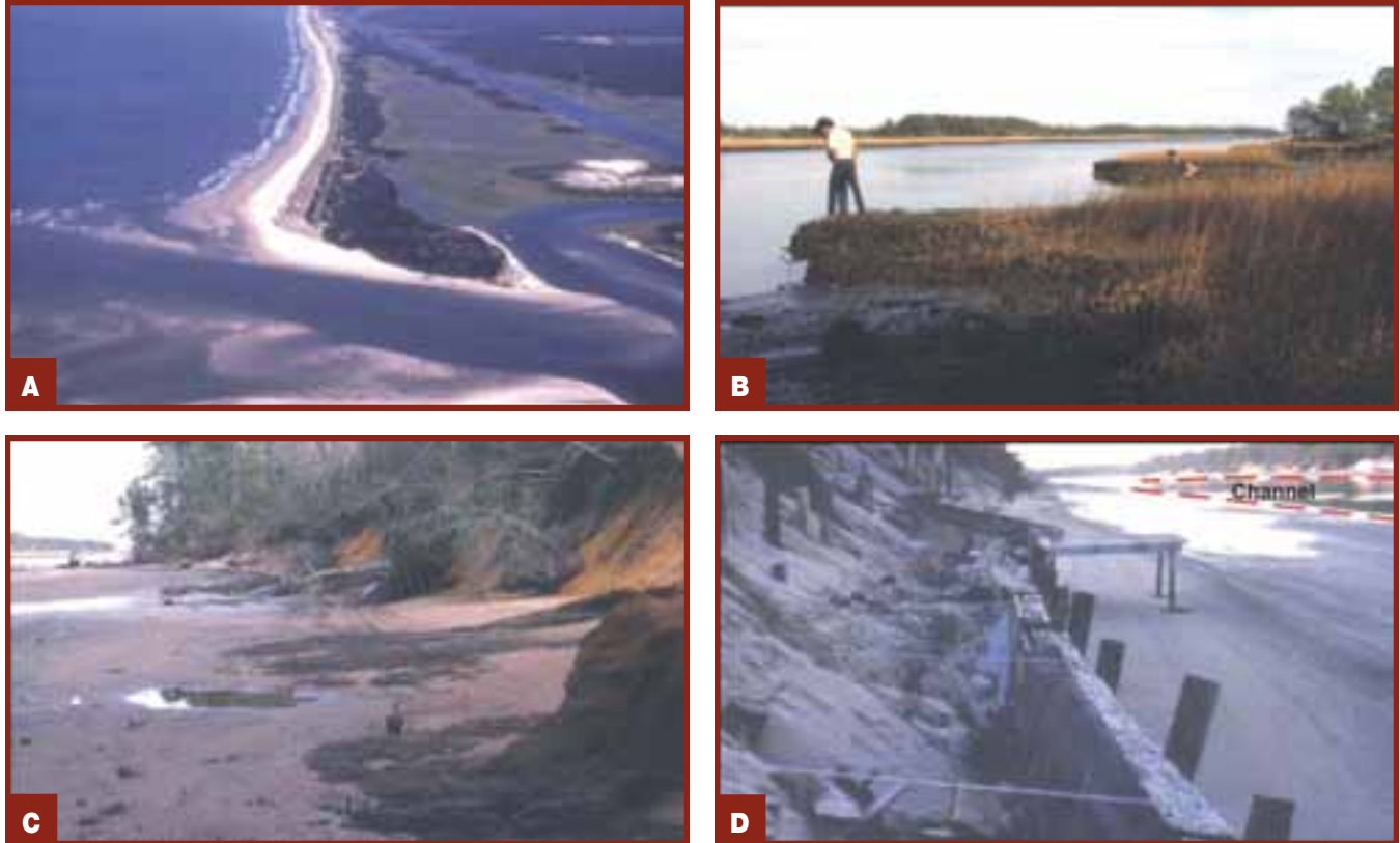
FIGURE 3-3-4. Photographs of shoreline erosion along the Intracoastal Waterway (ICWW) channel. PANEL A. Oblique aerial photograph of the east side of Onslow Beach and Browns Inlet in Figure 3-3-3 showing the ICWW cutting through the estuarine marsh (light green-colored vegetation) behind Onslow Beach in the foreground and the Pleistocene subaerial headland (dark green-colored vegetation) in the background. Notice the string of old, high and circular dredge spoil piles and the active, irregular-shaped dredge disposal site along the left side of the ICWW and covered with upland vegetation (dark green-colored). PANEL B. Photograph of the eroding estuarine marsh shoreline along the ICWW at low astronomical tide. Notice that at this tide level, boat wakes will erode the soft peat beneath the tough modern marsh root mass, producing a severe undercut peat block that will ultimately break off. PANEL C. Photograph of an eroding low to high sediment bank shoreline along the ICWW at low astronomical tide. Shoreline erosion will not take place during this tide level as the wave energy is expended on the very broad strandplain beach. However, during high tide, the boat wakes break directly on the base of the wave-cut cliff, severely eroding the bank with the ultimate failure of large slump blocks and associated trees. Notice the Pleistocene iron-cemented sandstone in the foreground that is slightly more resistant to the erosional process. PANEL D. Photograph similar to Panel C with a desperate, but unsuccessful effort to stop the erosional process. Assuming that the steps in the background are four feet wide, this shoreline has receded approximately 100 feet since the ICWW was cut in the 1930s, resulting in an erosion rate of about 1 to 2 feet per year.
