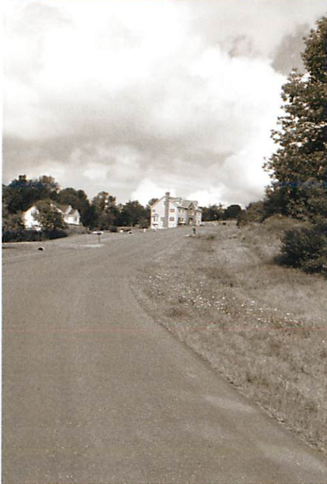
Breezy Knoll subdivision incorporates many “low impact” design elements, like a narrow paved roadway and engineered grass swales replacing traditional curb-and-gutter drainage.
