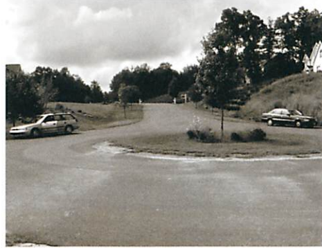
Innovative design can help reduce the impacts of impervious surfaces on water resources. (Lower left photo) A town road with reduced pavement width and curbless roads. (Above) A cul-de-sac with a vegetated center island in the Joshua Town subdivision.
