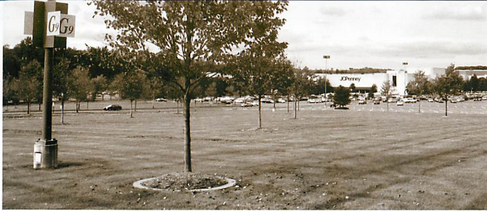
One solution to the problem of too much parking: Westfarms Mall in West Hartford and Farmington features an engineered grass overflow parking lot, to promote infiltration of stormwater.
