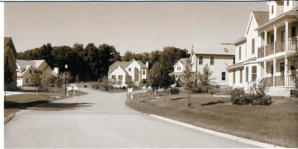
The transition from the conventional subdivision to the “low impact” subdivision at the Jordan Cove Project is marked by the change in the road surface from asphalt and curbs to pavers and grass swales.
