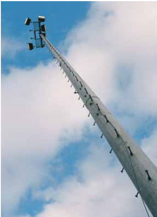
High mast lights mounted on 110 foot towers, in Valdez Harbor, Alaska. This tower has six 1,000 watt high pressure sodium light fixtures.
