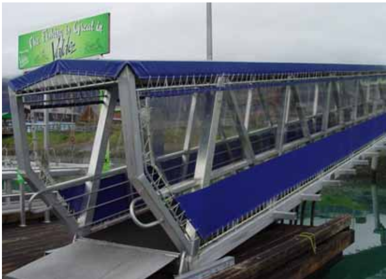
The cover on this gangway shields the walking surface from rain and snow.
