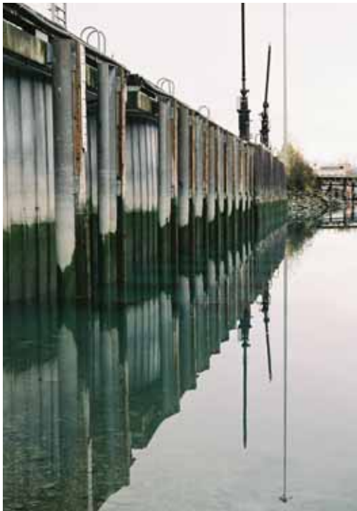
Galvanized sheet pile docks, like this one in Valdez Harbor, Alaska, have remarkable longevity in cold Alaska waters.
