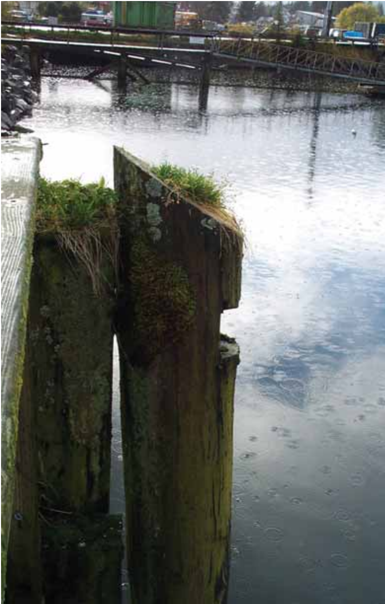
Wooden fender pile showing failure due to rot. While it is commonly thought that an angled cut helps shed water, this practice works against you by increasing the surface area.
