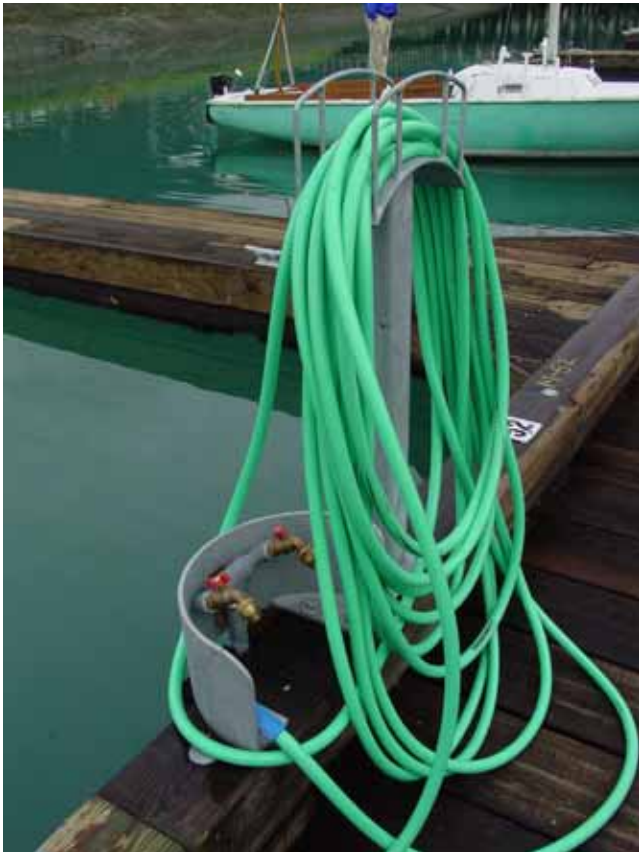
The convenient hose hanger, for the potable water system in Valdez Harbor, Alaska, was designed by Tryck, Nyman, Hayes, Inc.
