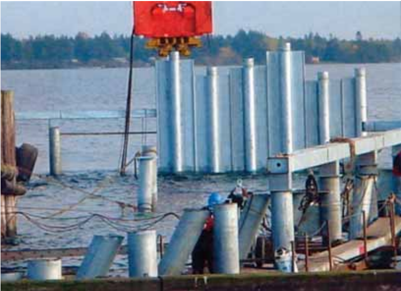
A sheet pile wave barrier, showing round steel piling with a section of sheet piling welded along its length on two sides, in Blaine, Washington.
