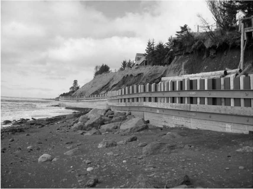
Figure 5. Bulkhead at Oceanic Bluff, Homer, Alaska.
