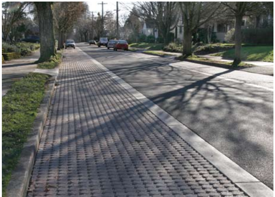
This pervious parking strip in Portland is one example of low impact design. Image © Bureau of Environmental Services, Portland, Oregon.
