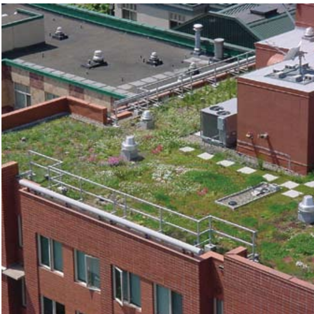
More examples of low impact design. Left: eco-roof planted with sod. Right: flow-through planters. Images © Bureau of Environmental Services, Portland, Oregon.
