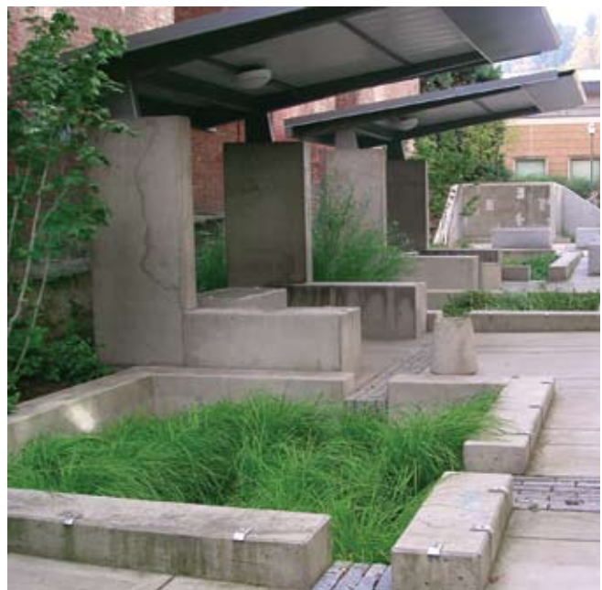
More examples of low impact design. Left: eco-roof planted with sod. Right: flow-through planters. Images © Bureau of Environmental Services, Portland, Oregon.
