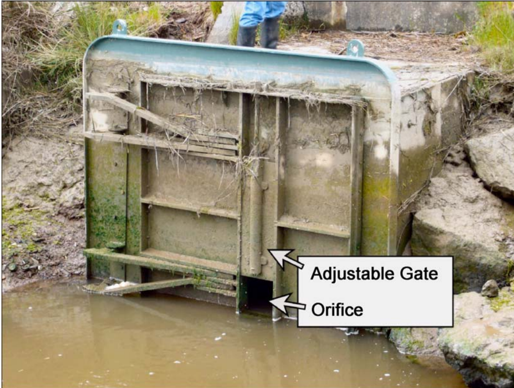
Plate 2. Side-hinged tide gate with adjustable orifice.
