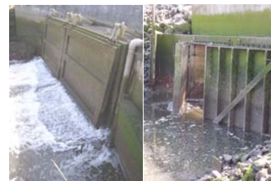
Figure 2. Before (l) and after (r) tide gates at Larson Slough, Coos Bay, Oregon.
