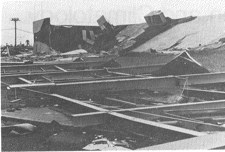
Fig. 2. The remains of a building after the walls were collapsed by winds of Hurricane Celia. Photo courtesy of the Texas Highway Department.
