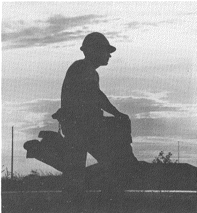
Fig. 33. A weary electric power line crewman takes a break during the recovery period from Hurricane Carla, September 1961, at Bay City. Photo courtesy of the Texas Highway Department.
