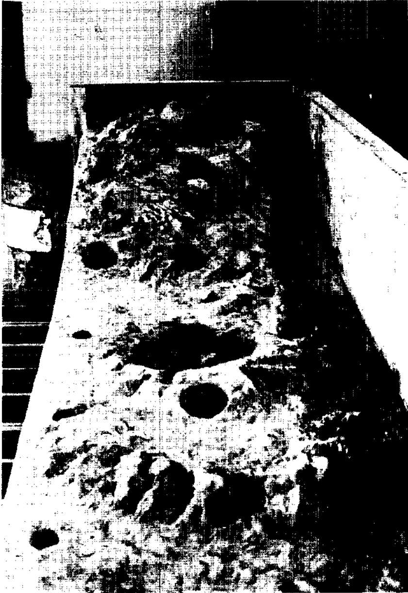
Figure 15. Tremie-placed concrete at completion of coring program. This sample is Test 1. Note core holes.
