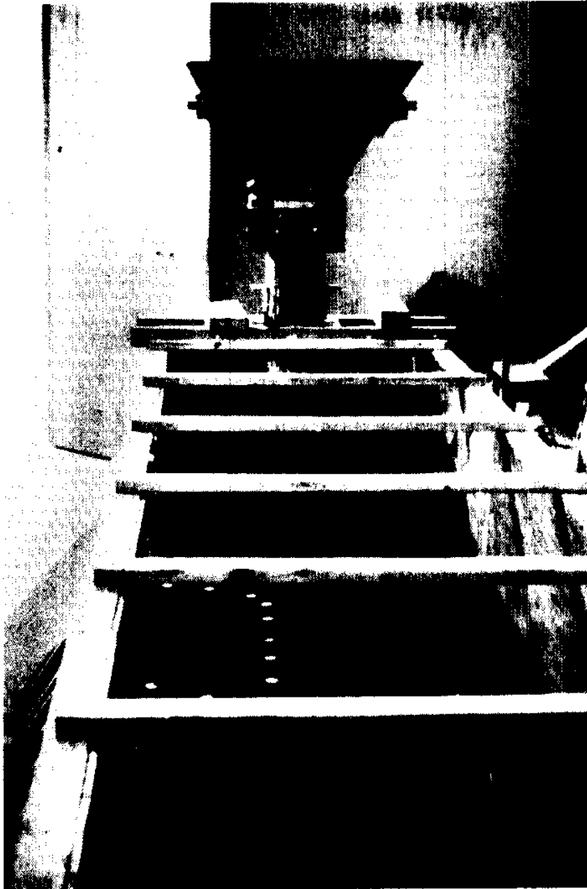
Figure 9. Tremie placement box completely assembled and ready for placement.
