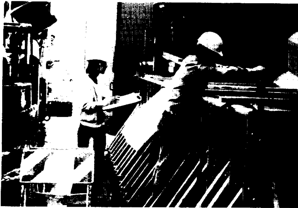
Figure 13. Taking soundings during break in concrete placement.
