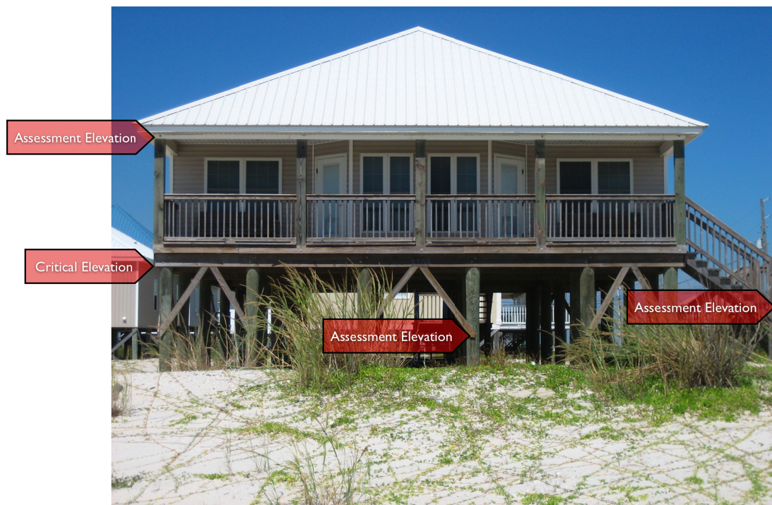
Figure 5. Example of subject structure photo showing locations of critical and assessment elevations included in the structural monitoring database.
