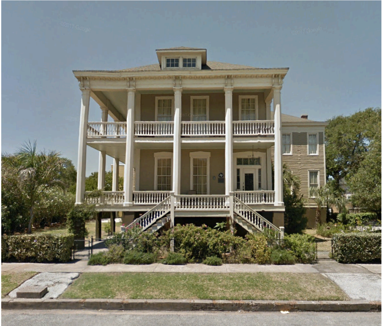
Figure 23. Lasker Home for Homeless Children is a Greek Revival style building on the National Register of Historic Places. Although it is out of the current 100-year floodplain, it will be within the 50-year floodplain in 2050 and the 25-year floodplain in 2100 if the intermediate-high sea-level rise scenario verifies.
