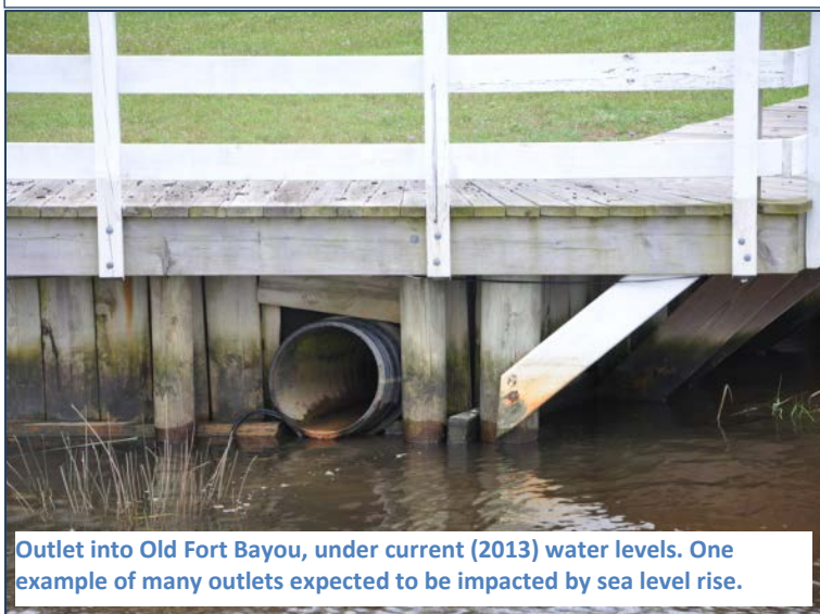
Figure 5.3 Stormwater Outlet into Old Fort Bayou
