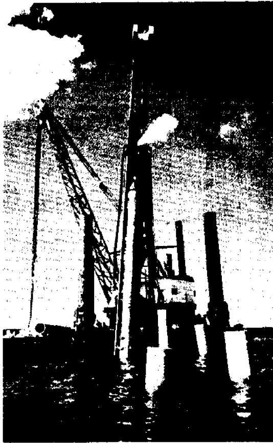
a) Driving Piles
