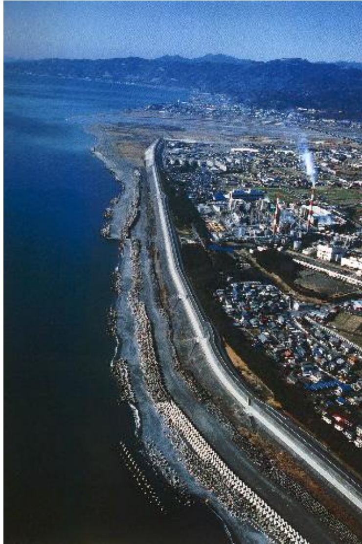
Figure 1.2: Several rows of wave absorbing breakwaters in front of seawall (17 m above sea level) constructed on Fuji Coast in Japan to reduce wave overtopping and beach erosion (Japan Society of Civil Engineers, Committee on Coastal Engineering 1994)
