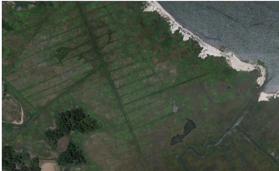
Figure 2.3: Satellite image showing an example of the artificial, man-made ditches, called "mosquito ditches," in the upper Brockonbridge Marsh ( Imagery courtesy of Google Earth )
