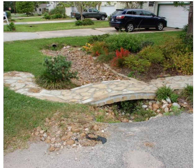
Existing drainage swale on private property
