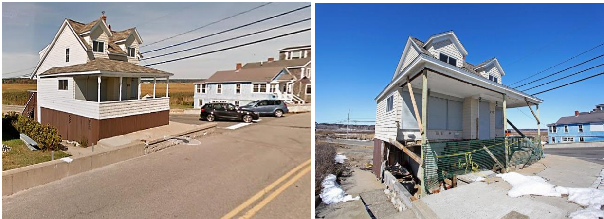
Figure 6: Image on Left Shows House Before Norester (Google Maps) Image on Right is the Same House After Nor'easter (Buttarazzi)
