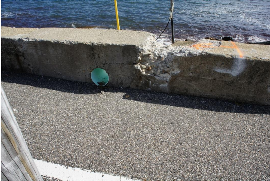
Weep hole through seawall along Webhannet Drive
