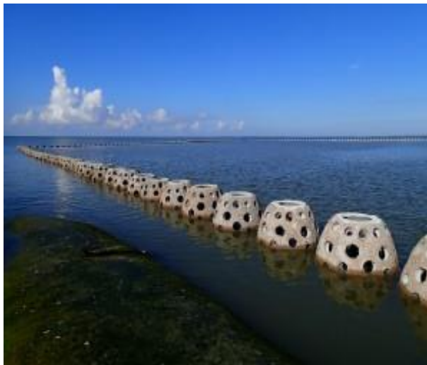
Figure 14: Reef Balls in Use Along the coast of Texas (Reef Ball Foundation)
