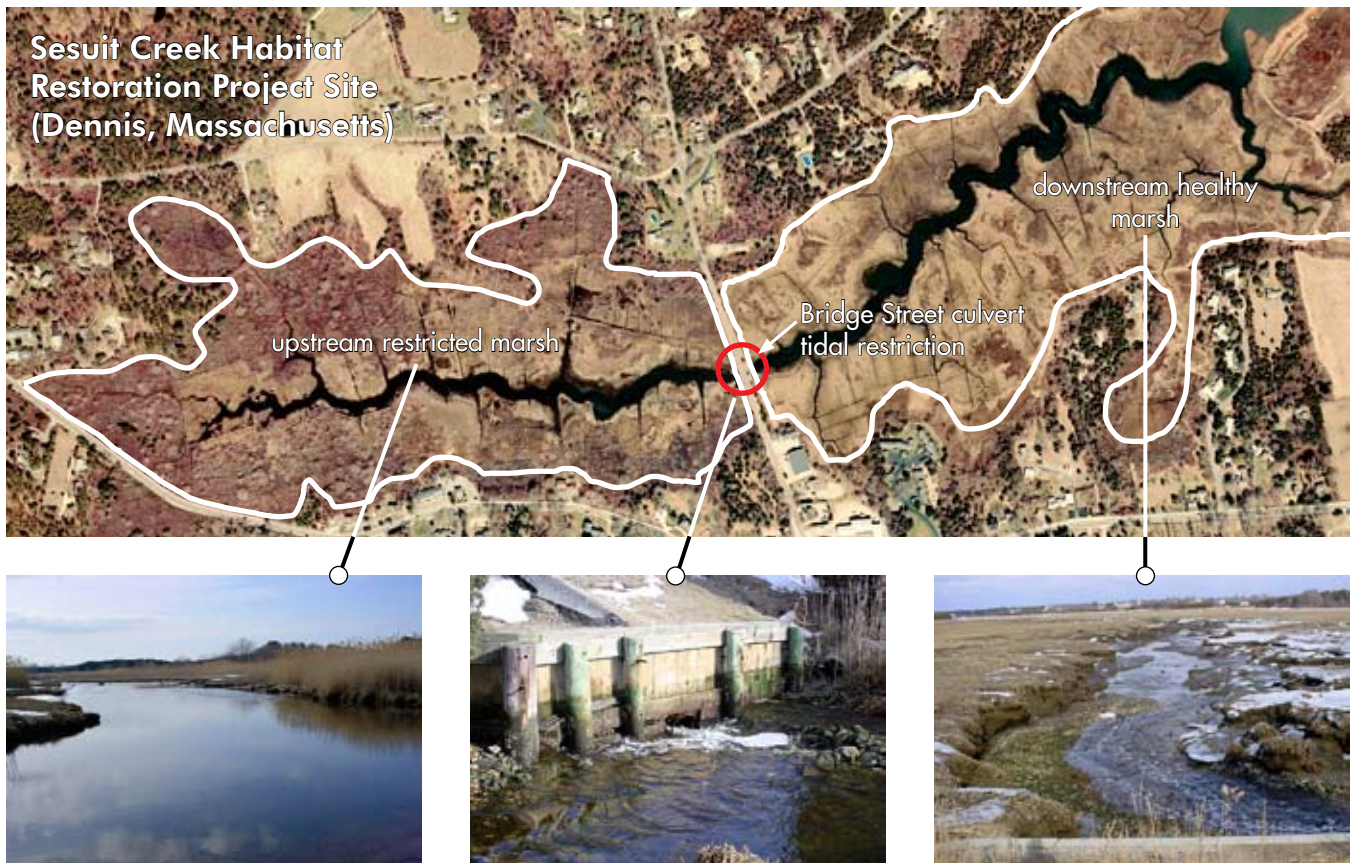
An aerial photo (top) shows the location of a culvert under Bridge Street in Dennis, Massachusetts. The culvert restricts tidal flow into the marsh area to the left, affecting the environmental conditions and types of plants living there. Differences in vegetation make the restricted and unrestricted areas have different colors in this aerial view. Three ground-level photos show the restricted marsh (left), Bridge Street culvert (center), and unrestricted marsh (right). Massachusetts Office of Coastal Zone Management
