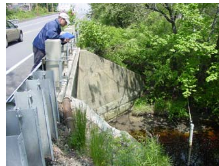
Figure 17. Webhannet River at US Route 1. Sewer line crossing bridge.
