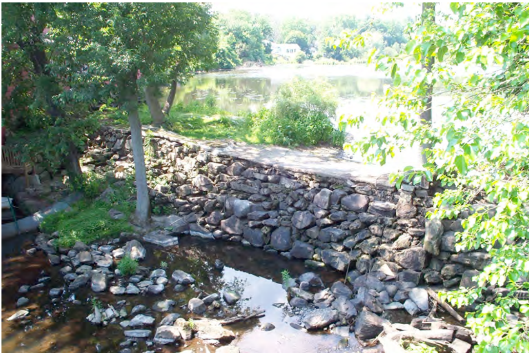
Figure 2. Example of migratory barrier, photo credit CTDEP/Inland Fisheries Division.
