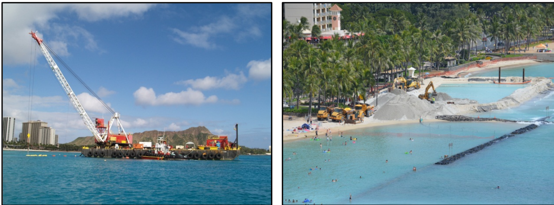
FIGURE 7: Sand recovery barge and dewatering basin
