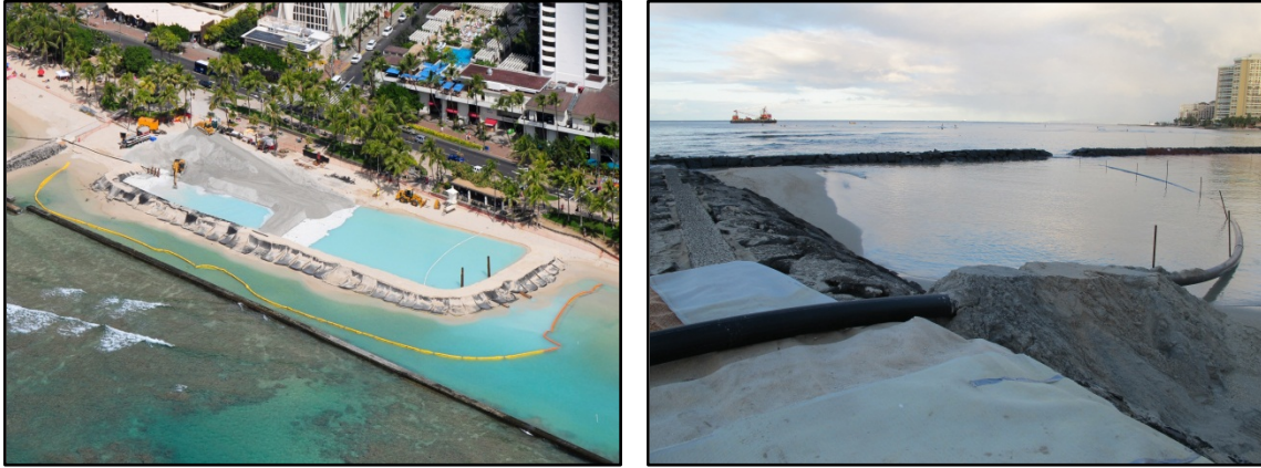
FIGURE 8: Dewatering basin (left) and sand recovery pipeline (right)
