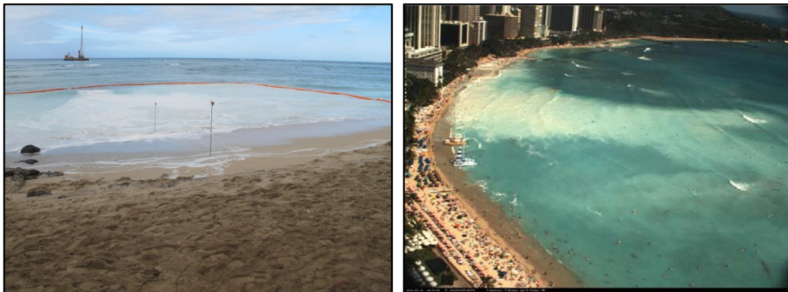
FIGURE 13: Sediment plume formed despite the use of containment booms
