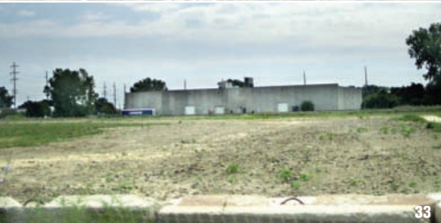
Before: Manufacturing activities contributed to polychlorinated biphenyl (PCB) and other contamination at brownfield site.
