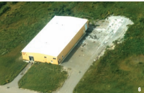
Before: Parcel with a vacant building and contamination from semi-volatile compounds and heavy metals.
