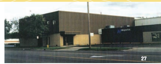
Before: Site contaminated with petroleum and chlorinated solvents; given to the city of Owosso in 1996.
