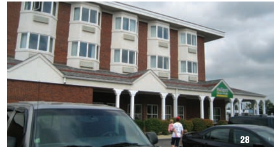
After: Remediation and redevelopment resulted in the development of the Comstock Inn and Mulligan's Irish Pub.
