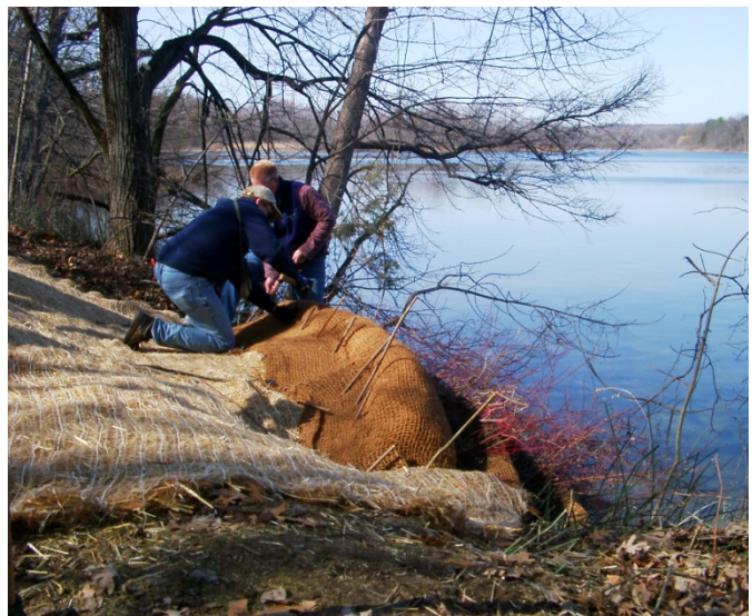
Figure 13. Stabilizing the shore of a lake in southern Michigan using natural materials and shrubs.
