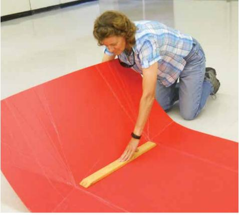
After bending the first folds, you can see where the corners of the inside rectangle are on the bottom side of the plastic.
