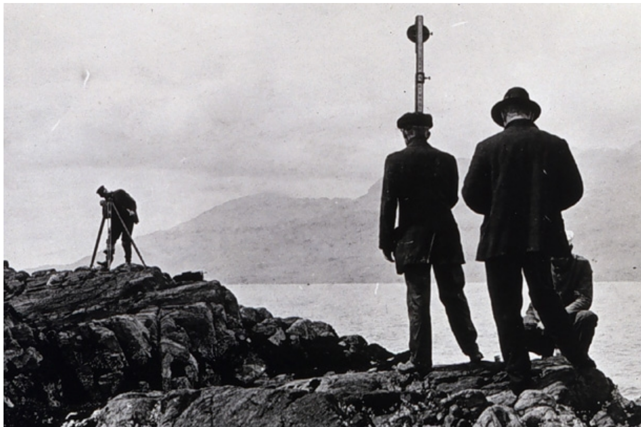
A U.S. Coast and Geodetic Survey work party calibrating a tide staff against a land-based benchmark on Cat Island, Southeast Alaska in 1915. Original from NOAA Photo Library.
