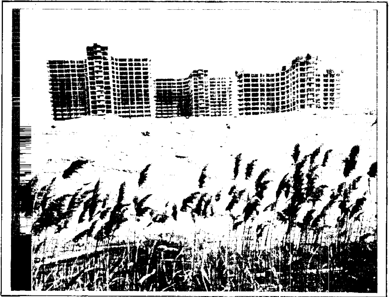
Coop City during construction. Pelham Bay marshland is seen in foreground.
