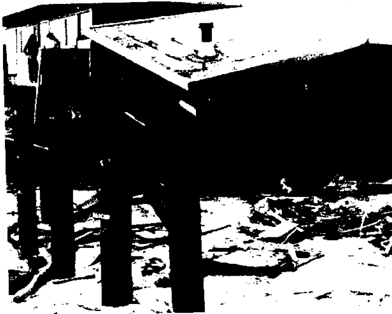
Figure 6. Collapse of a home built on shallow pilings on Rio del Mar Beach, Monterey Bay, during the winter of 1983 due to beach scour.
