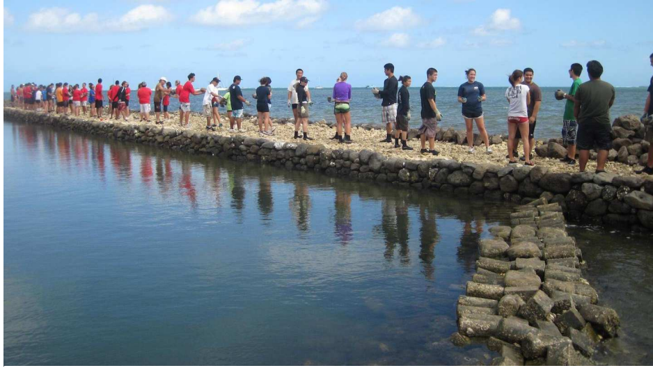
Figure 7: Wall restoration project at He'eia. Photo Credits: Paepae o He'eia
