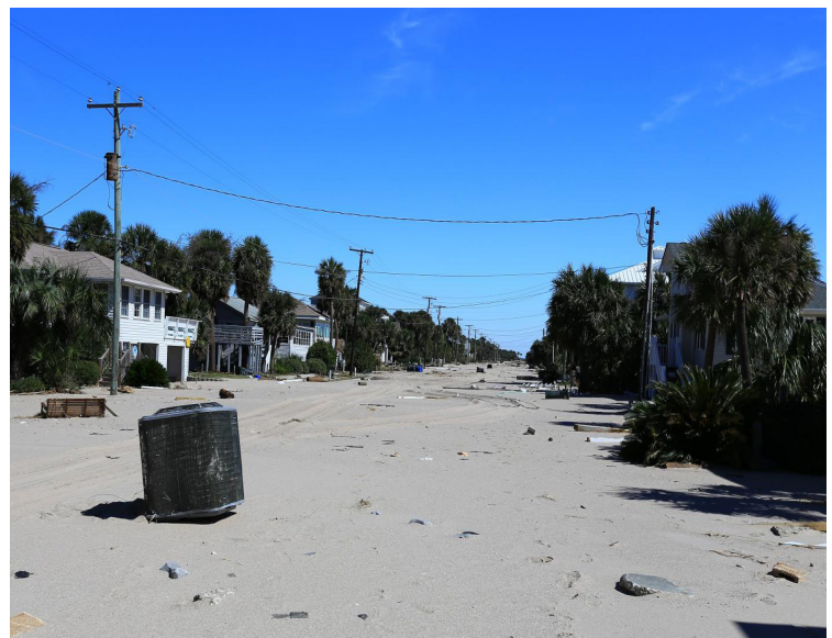
Figure 2.3 Air-conditioning unit sits on S.C. Highway 174 on top of a layer of sand deposited by Hurricane Matthew. Edisto Beach, S.C. National Weather Service, NOAA (2016)
