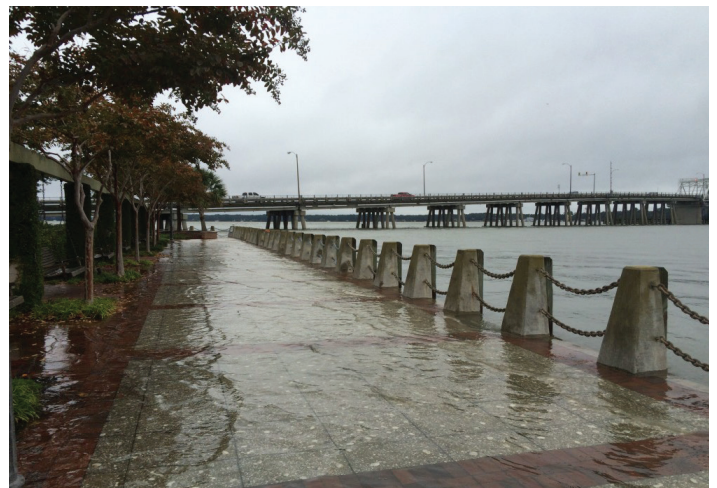
Figure 1.10 Tidal flooding along waterfront in Beaufort, S.C. Jeramie Stanley as reported to King Tide Report (October 27, 2015)
