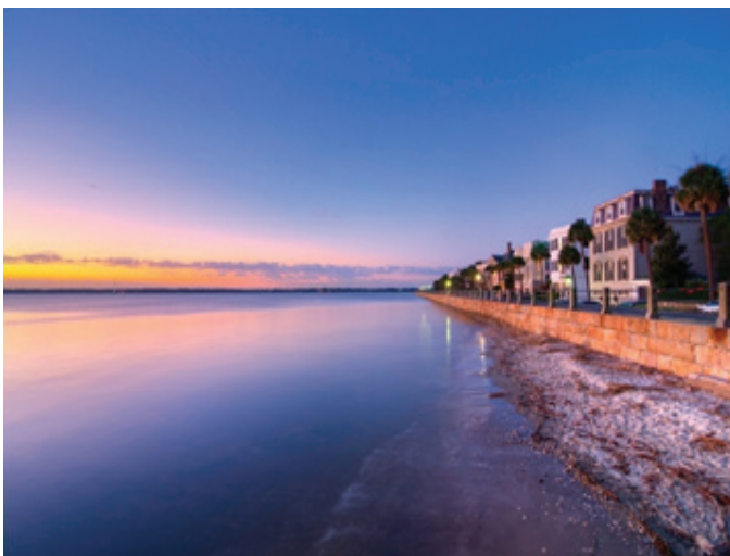
Figure 5.1 Eastern section of the Battery, a seawall in Charleston. S.C. Sea Grant Consortium.
