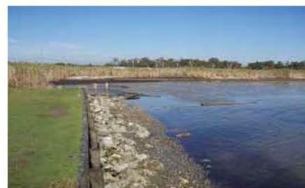
Figure 1. Substantially eroding shoreline, directly adjacent to a shoreline armored with a bulkhead and rip-rap.
