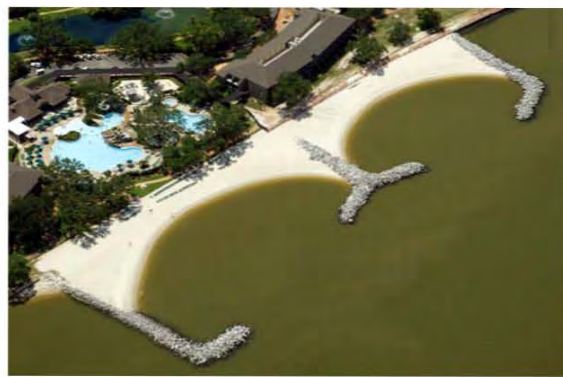
Figure 2. Photograph of an artificial beach on Mobile Bay stabilized by headland breakwaters
