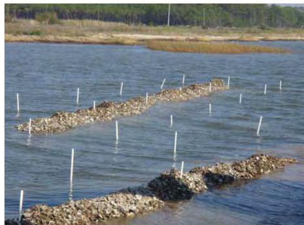
Figure 1: Photograph of one of the breakwater reef complex constructed near Bayfront Park, AL.
