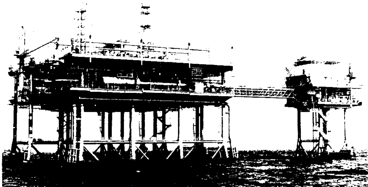
Figure VII-40. A supertanker ties up offshore to unload its crude oil through floating hoses into LOOP's offshore pumping platform. The pumping platform then moves the
