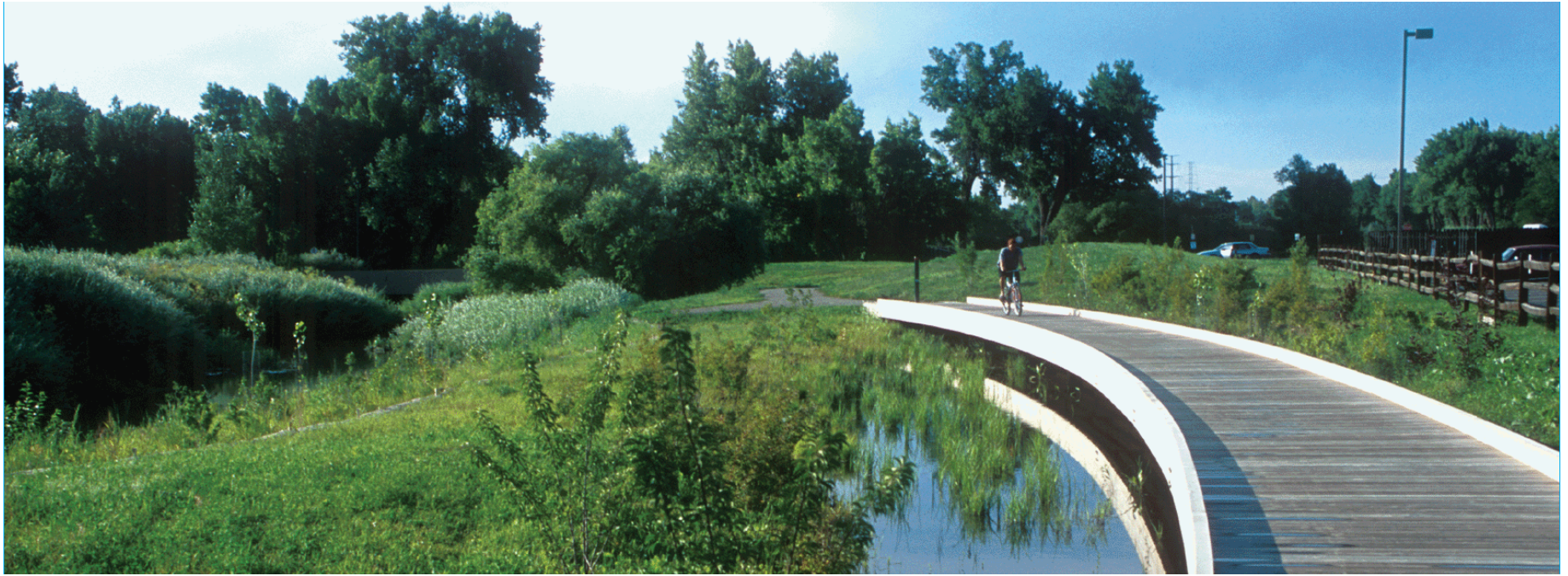
Photo: Multi-benefit park project with wetland treatment for parking lot runoff, recreational trail, and habitat enhancement in Denver, CO
