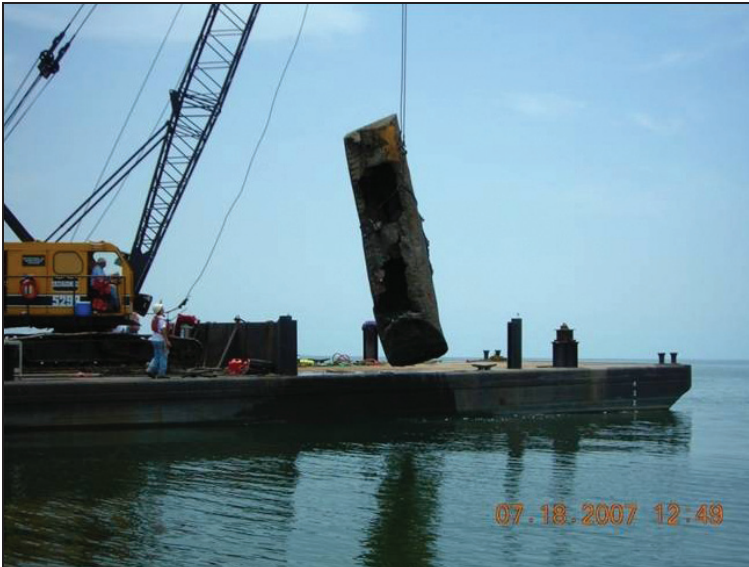
Figure 5: FEMA-funded removal, Mississippi. Photo: USCG
