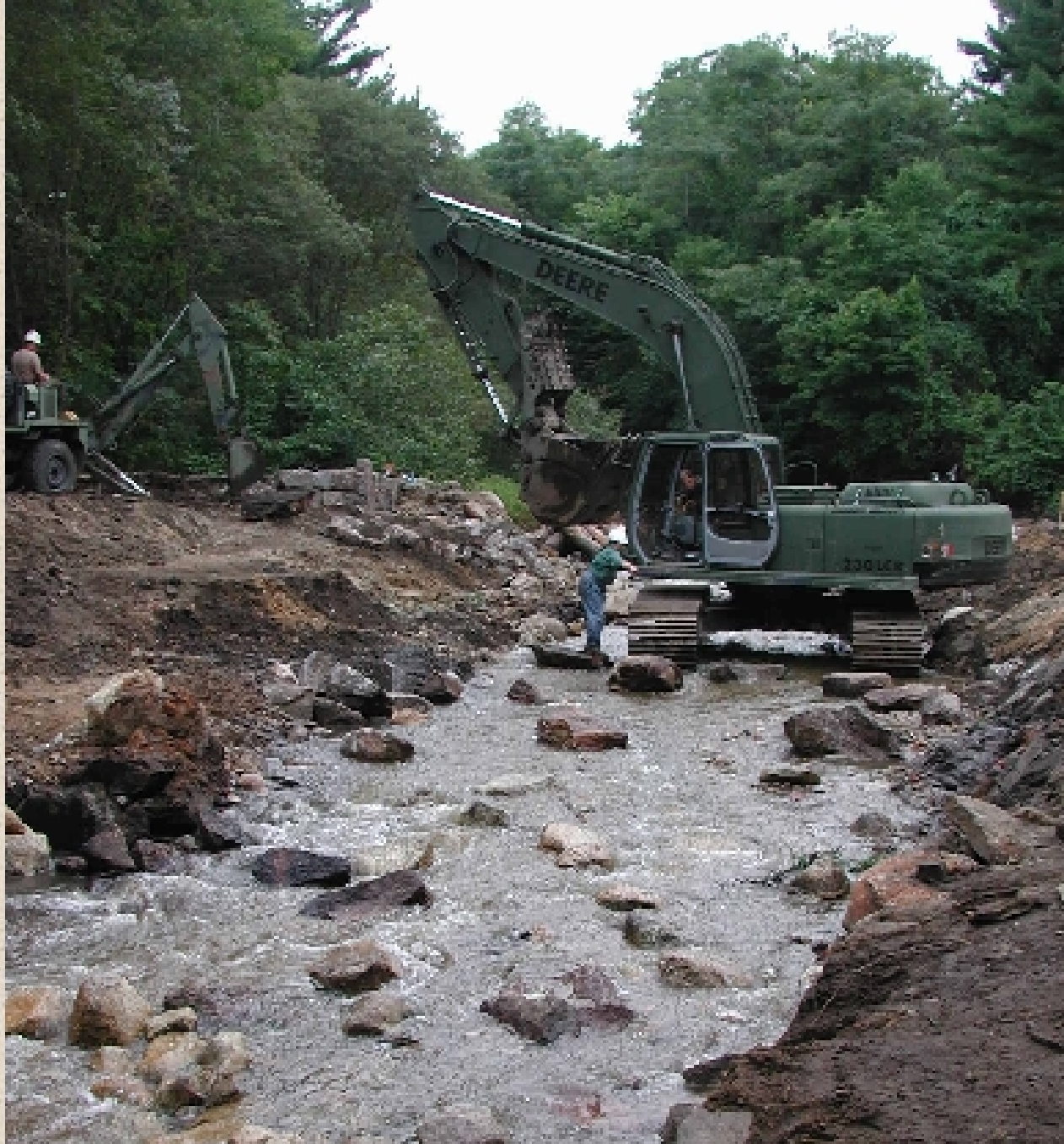
Massachusetts: Billington Street Dam Removal, Town Brook
