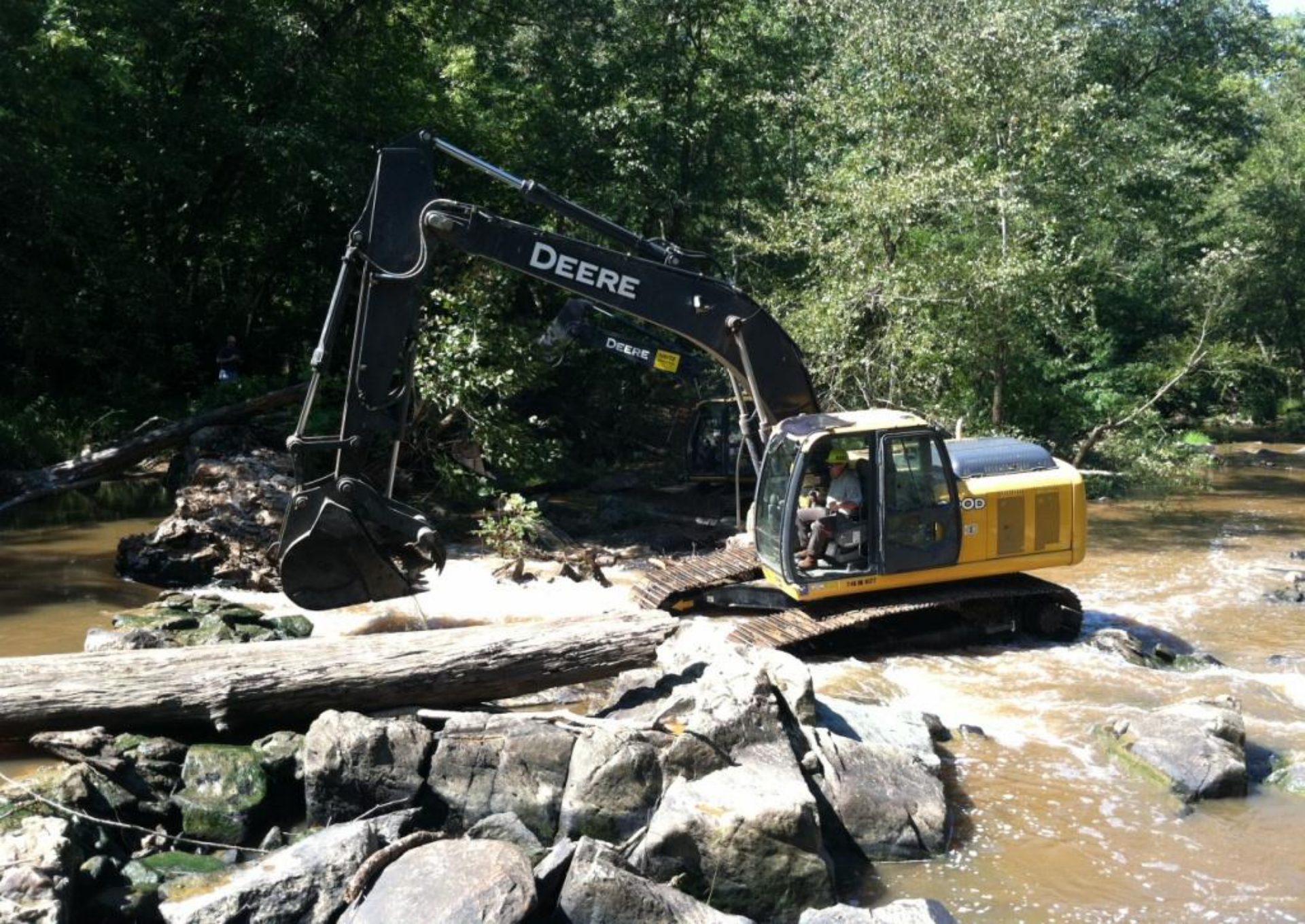
North Carolina: Dynamo Dam Removal, Little River
