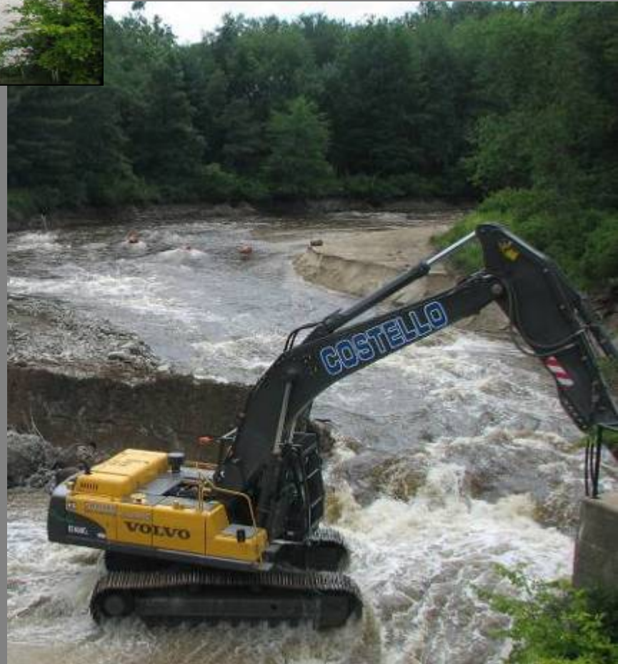
Merrimack Village Dam Souhegan River Merrimack, NH
