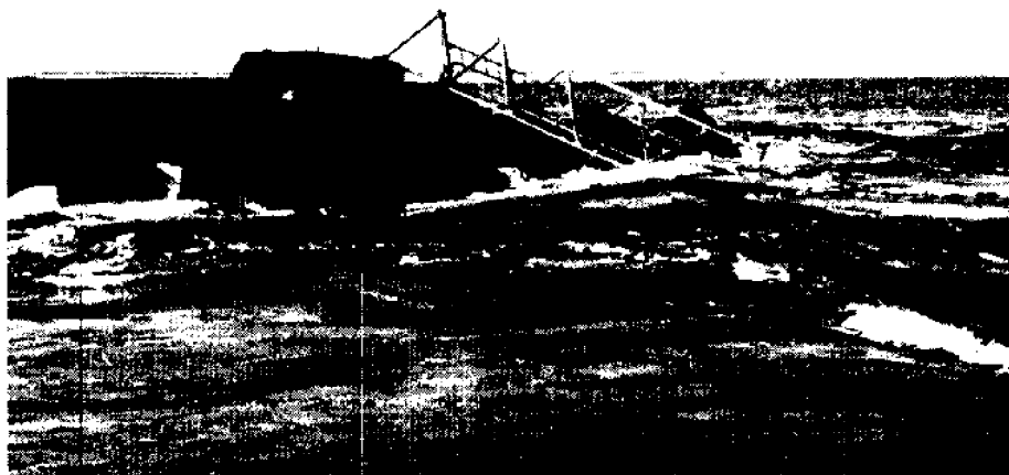
Figure 43 Deterioration of Tip of North Jetty and Fallen Light Tower
