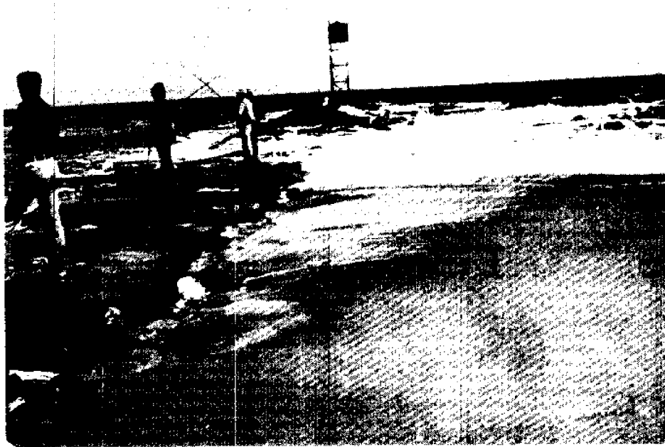
Figure 29 Sand Being Carried Over the South Jetty by Ocean Waves
