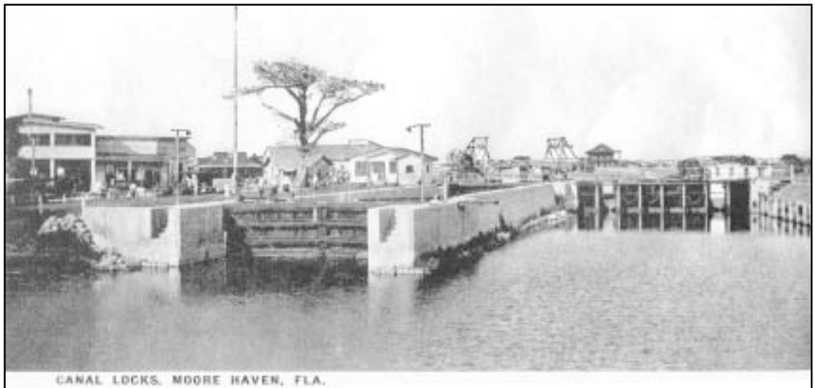
Figure 21b. Moore Haven lock.
