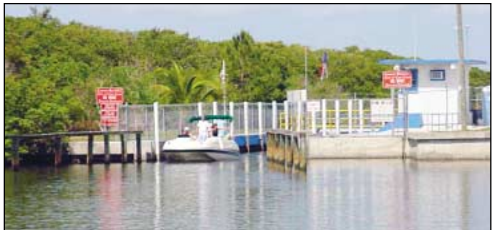
Lock at the entrance to the Cape Coral South Spreader Canal.
