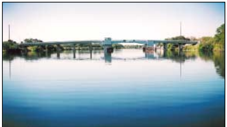
Figure 12b. Alva bridge, 2001.
