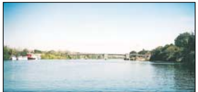
Figure 17d. La Belle bridge (now).
