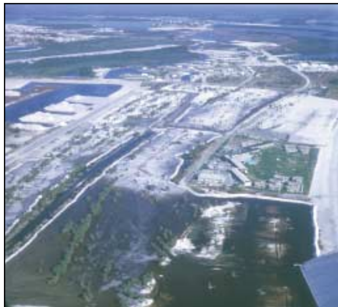
Aerial photograph of Marco Island under construction.
