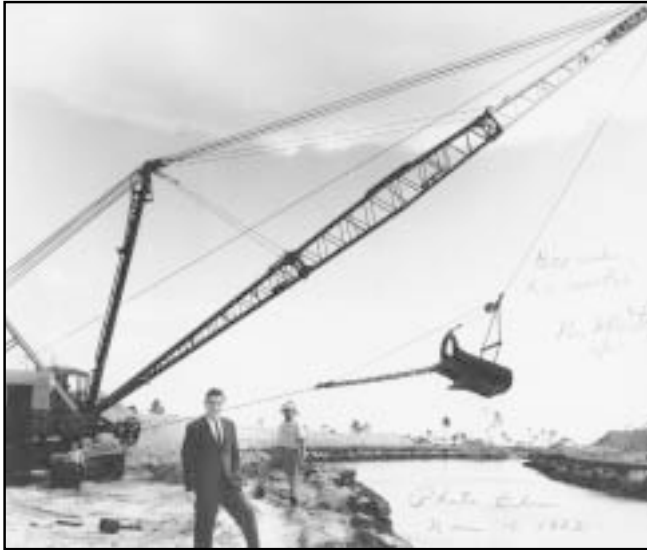
Figure 7. Dragline at Cape Coral, 1962.
