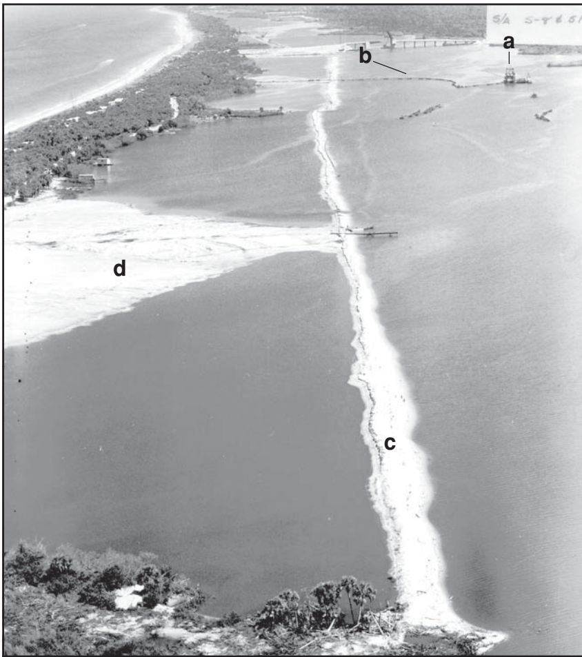
Figure 9. Dredge and dike
