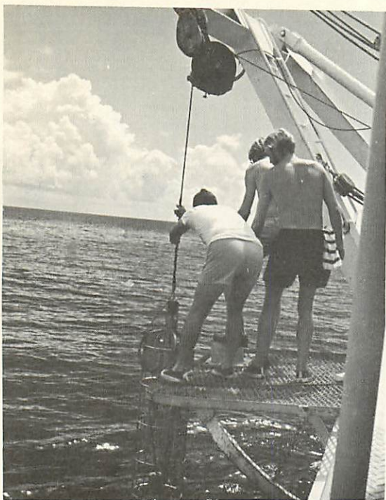
19. Students are exposed to modern equipment. They are lowering a S.T.D. (Salinity, Temperature and Depth) "fish."
