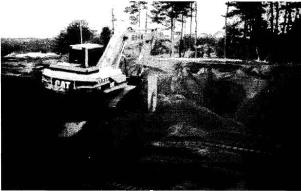
Figure 5. Burying Oiled Sand in Industrial Waste Dump
