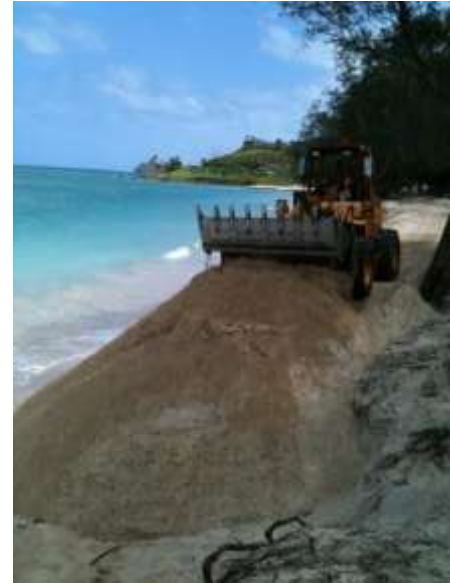
Dune restoration (sand back-passing) at Kailua, Oahu.
