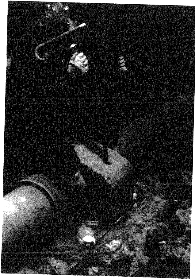
Diver installing concrete saddle to anchor Techite pipe.
