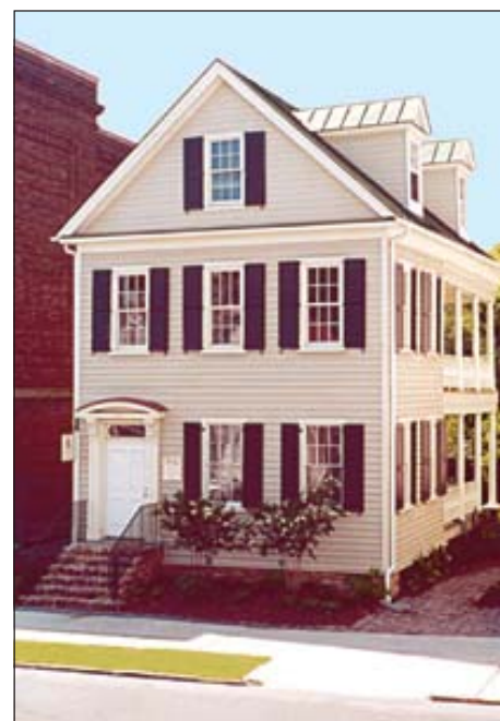
113 Calhoun Street: A Center for Sustainable Living
