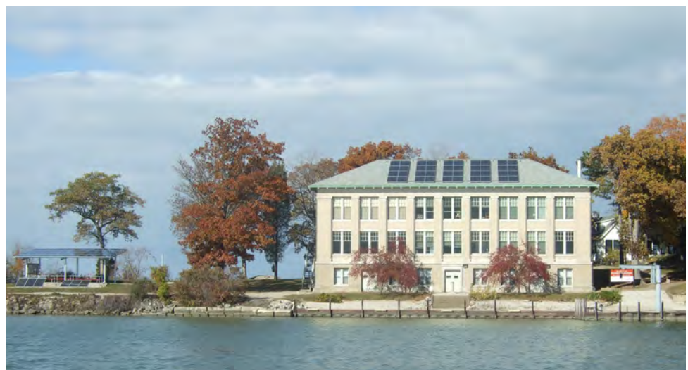
Renovations continue annually at Stone Lab. Most recently, 40 solar panels were added to the laboratory roof (above) and exterior enhancements to the Research Building were completed in 2013.
