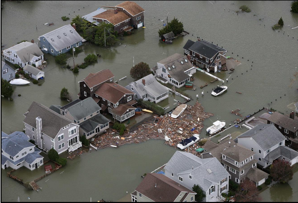
Hurricane Sandy Damage in Seaside, New Jersey, October 30, 2012 (T. Larsen/N.J. Governor's Office)
